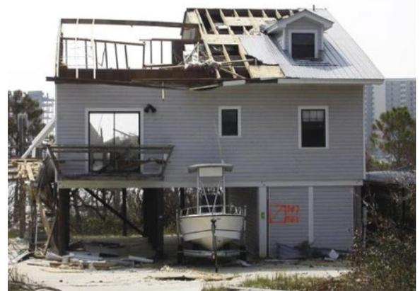
Figure 1: Severe damage to the roof framing during Hurricane Katrina.
